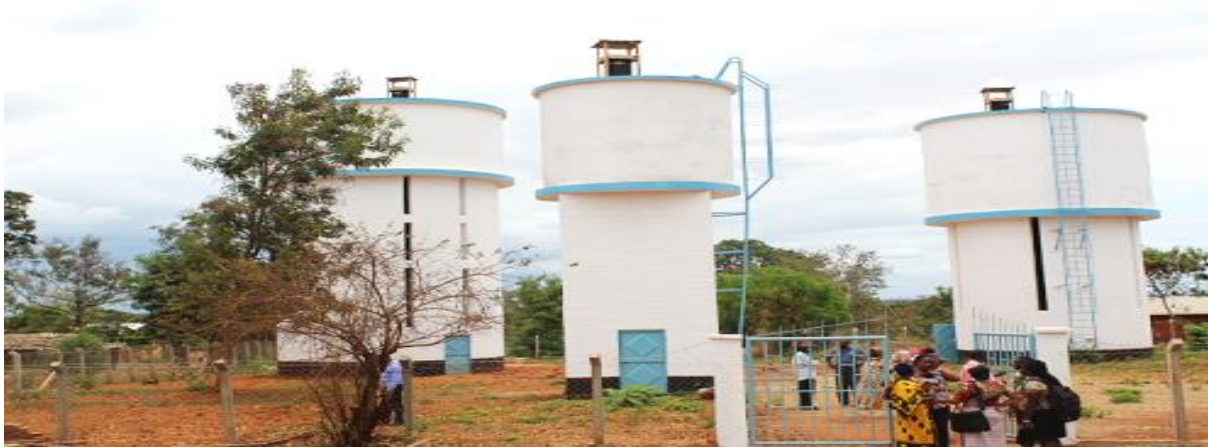
Water storage tanks constructed or rehabilitated by Water Resources Integration Development Initiative (WARIDI) at Msowero in Morogoro Region. Photo: WARIDI/ Yussuf Kajenje
