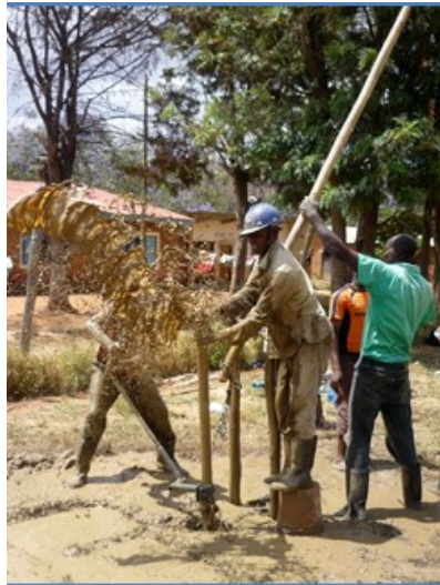
A Rota sludge team drilling a school borehole in Morogoro.
