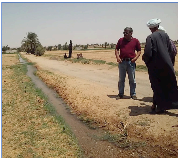
Much of the water in earthen canals — like the one seen here in the Qena governorate — is lost to seepage before it reaches the crops.
